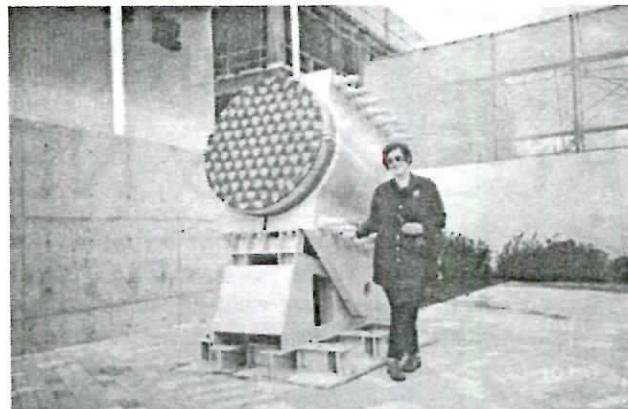
**Fig. 2:** The Akashi-Kaikyo Bridge, Leena Virola measuring The 1/1- scale model of the Ø 1122 mm main cable. Photo taken near the Maiko Pavilion, at Kobe side.
